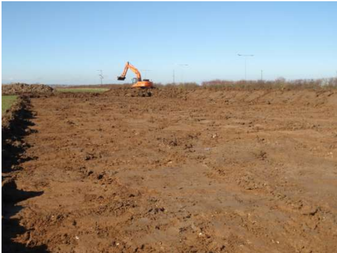
Plate 3. View of topsoil strip (looking west)
