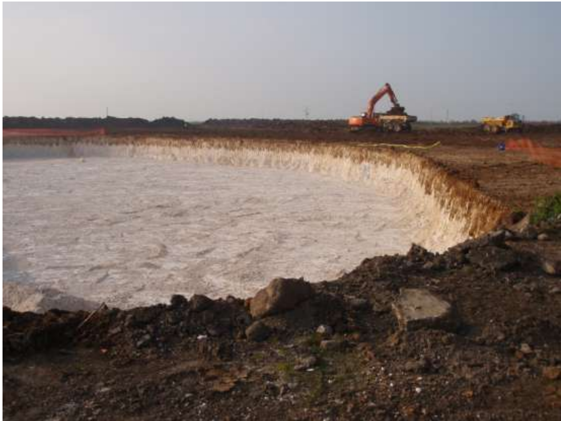
Plate 4. View of ground reduction
